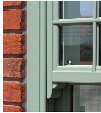
Run through sash horns
